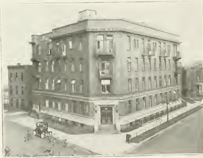
Sarah Morris Hospital for Children is one of the most attractive medical foundations in Chicago. It was built in connection with Michael Reese Hospital under a liberal agreement whereby the children of the donor were given authority to determine the object to which the funds should be devoted.
